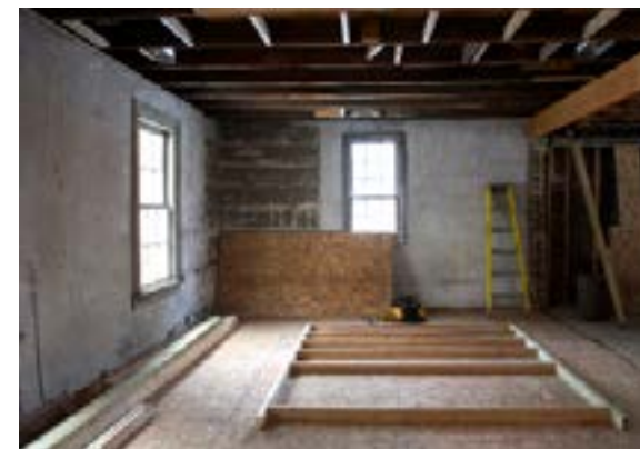
CONSTRUCTION OF WALL AND SUBFLOOR IN 1848 KITCHEN AND LARDER
