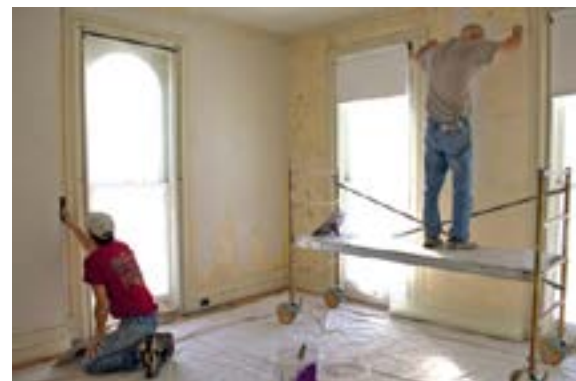
SCHROCK PLASTERING IN THE WEST WING
